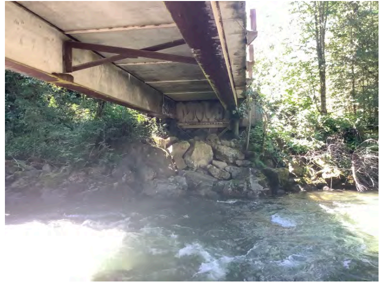
Left Bank Abutment when facing downstream
