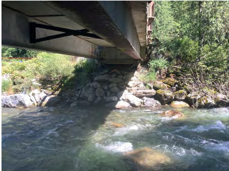
Right Bank Abutment when facing downstream
